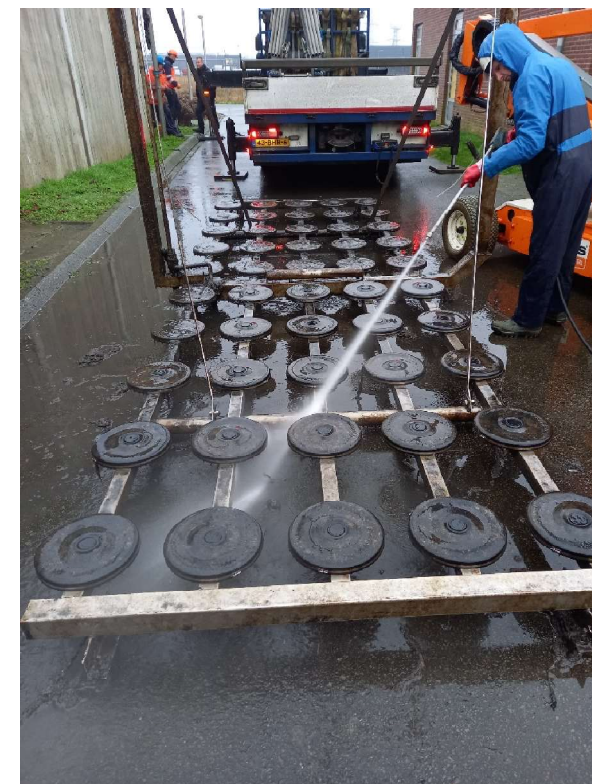
Cleaning of the diffusers
