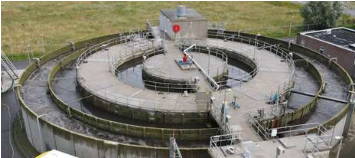
Normal aeration of outer ring with all aeration elements
