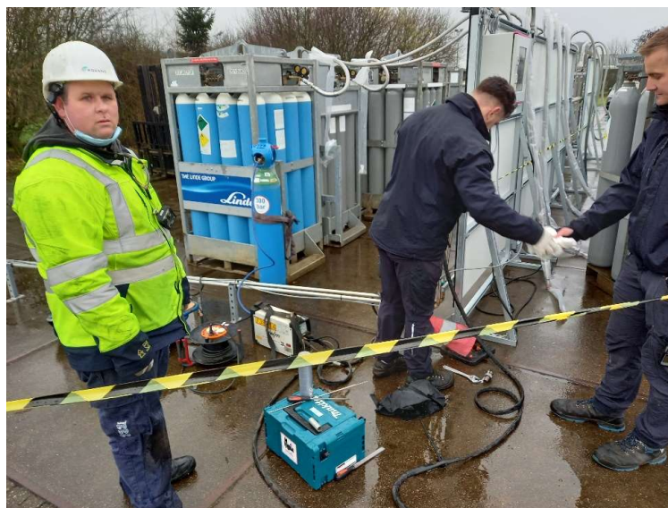
Last minute repairs at PO supply
